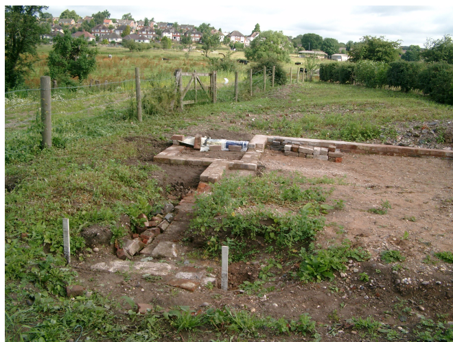
Lock House site looking north.
