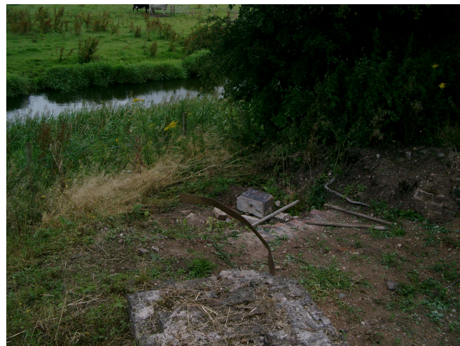
The end of the channel which led to the aqueduct and then the Lock.
