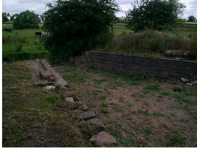
The north part of the Basin showing the channel which led to the aqueduct.
